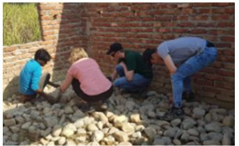
We undertook some building works. Here we are placing small boulders onto the ground side by side, water is then added. The rocks are then rammed into the ground to provide a firm support. Dirt mixed with cow dung helps seal it from water on the top or if they can afford it—a small concrete layer.
